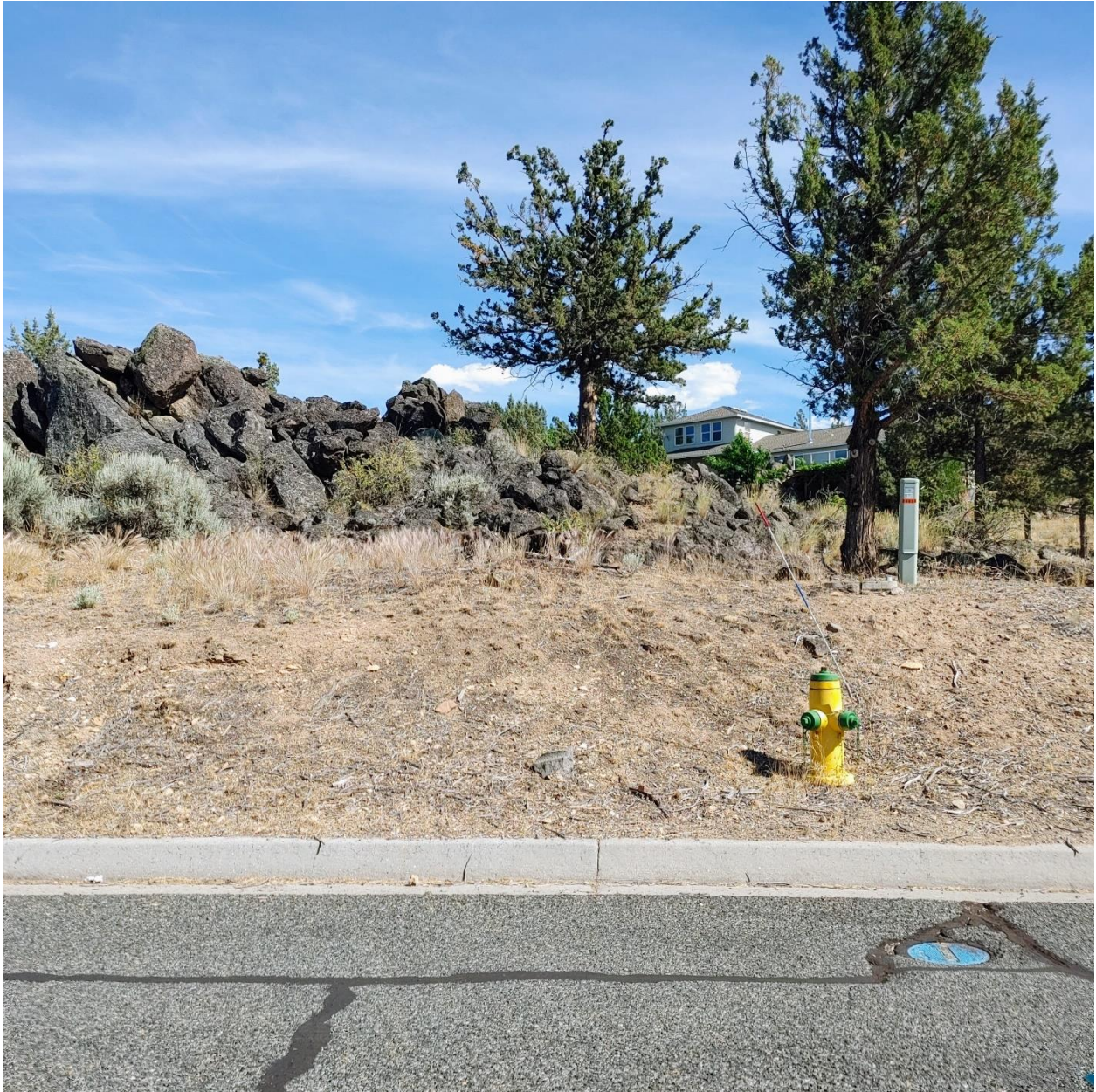
Photo 7: Looking east from Mountain Wood Drive onto fire hydrant #275 that will be replaced with a new fire hydrant. This fire hydrant is surrounded by asphalt, large rocks, gravelly soil, and juniper trees. The soil directly around the fire hydrant will be disturbed as all parts of the hydrant will be replaced down to the elbow in the ground.
