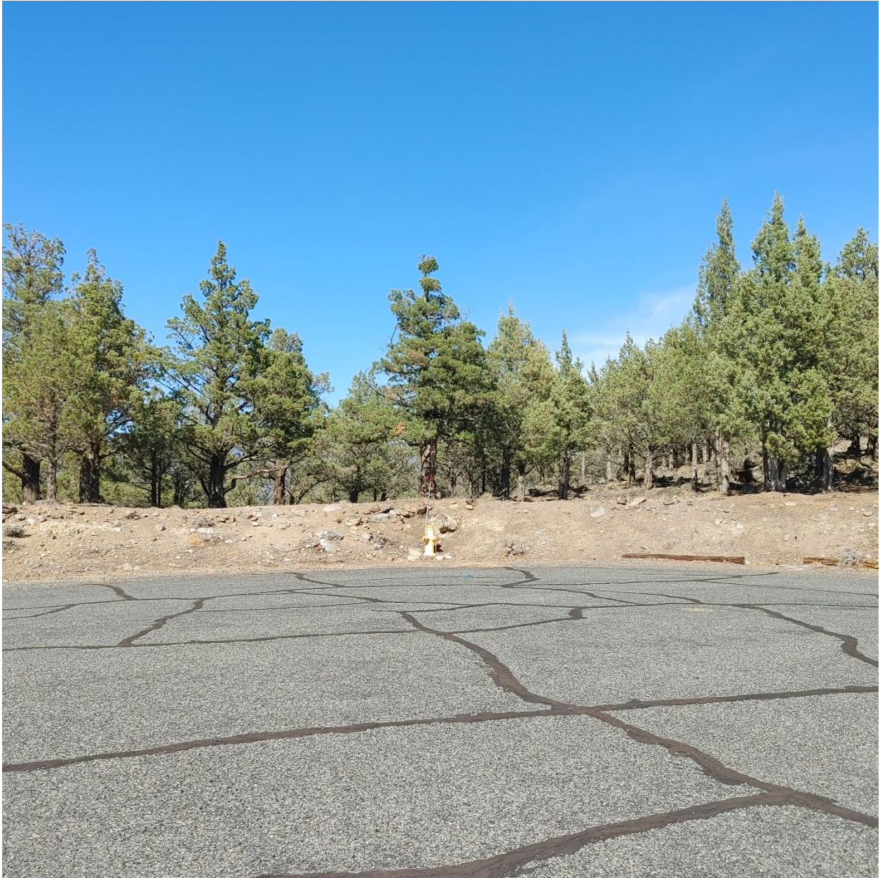
Photo 6: Looking North east from the cul-de-sac of Stone Crest Drive at fire hydrant #289 that will be replaced with a new fire hydrant. This fire hydrant is surrounded by asphalt, small rocks, gravelly soil, and juniper trees. The soil directly around the fire hydrant will be disturbed as all parts of the hydrant will be replaced down to the elbow in the ground.
