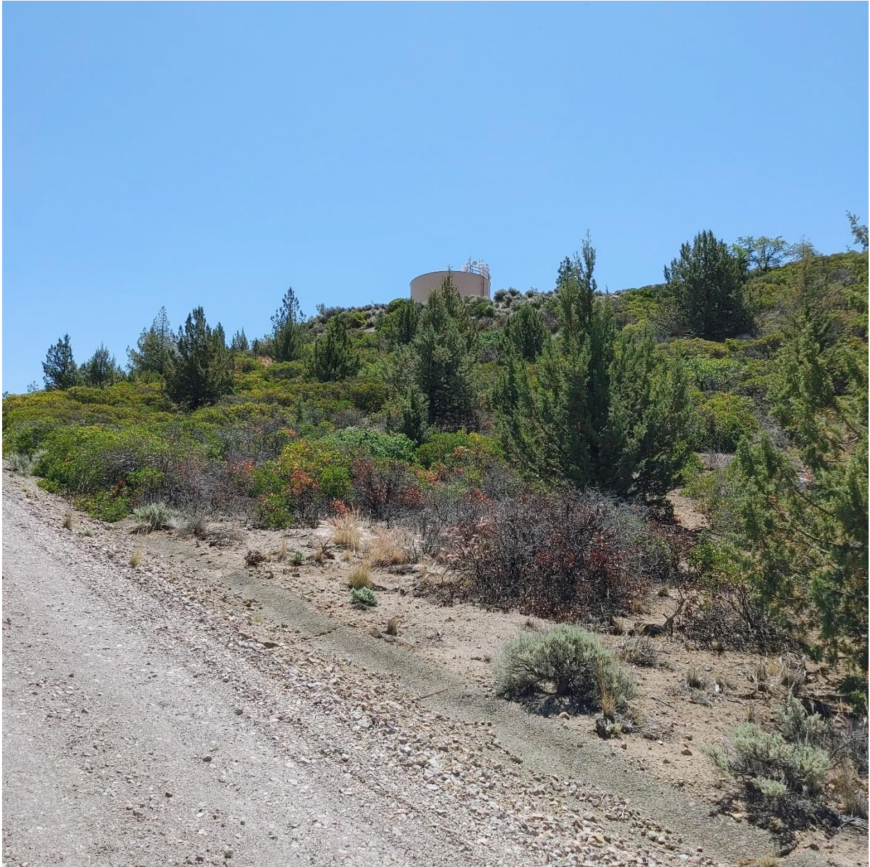
Photo 4: Looking south from the service road to water tank #4 that will be replaced with a larger water tank. Water tank #4 is surrounded by manzanita shrub, gravelly soil, and juniper.
