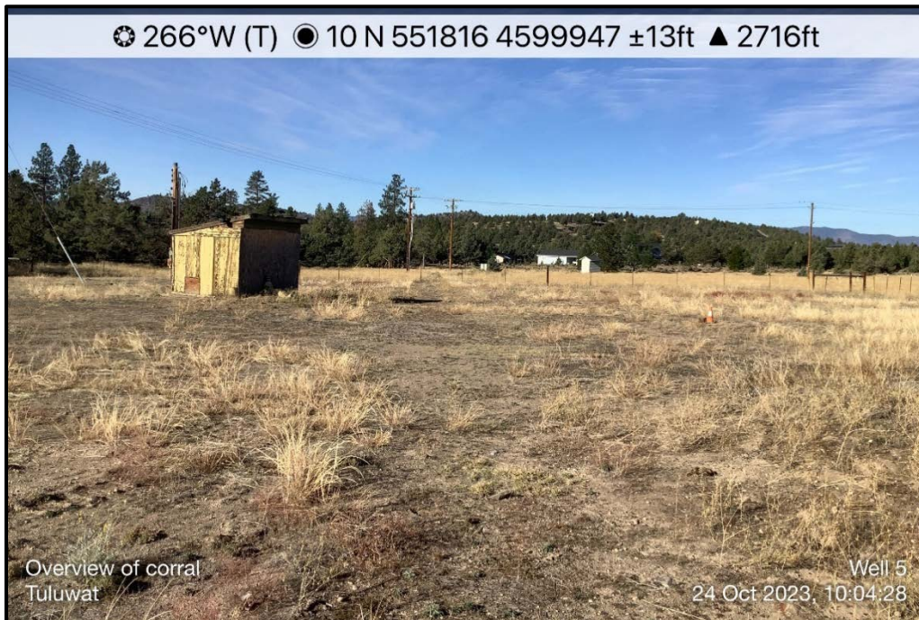
Figure 6. Well No. 5 and well house in a horse/cattle corral.
