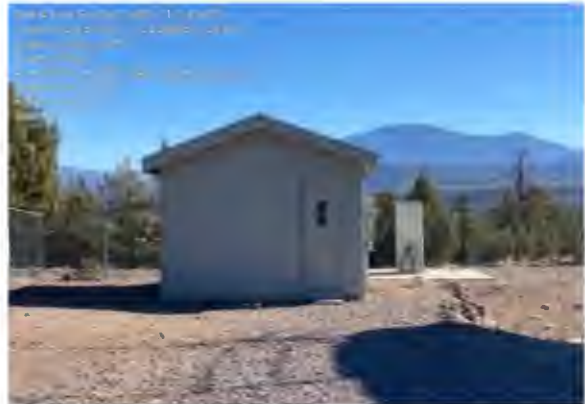
Photograph 3.8 Booster Pump Station B-50
