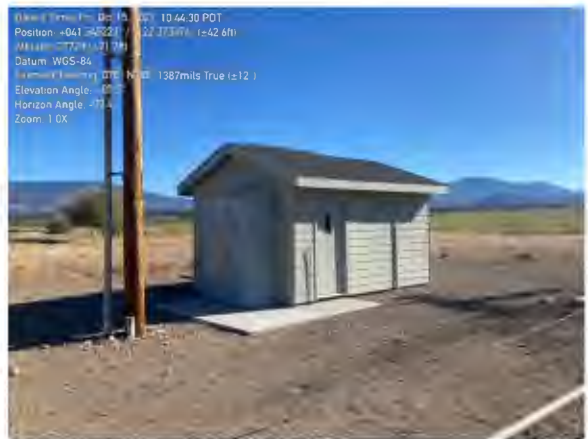
Photograph 3.1 Well #4 Well House
