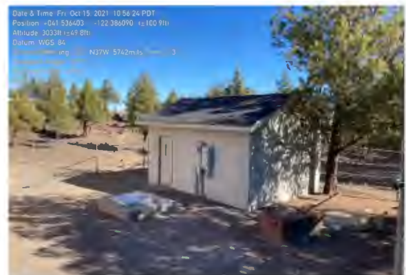
Photograph 3.10 Booster Pump Station B-56
