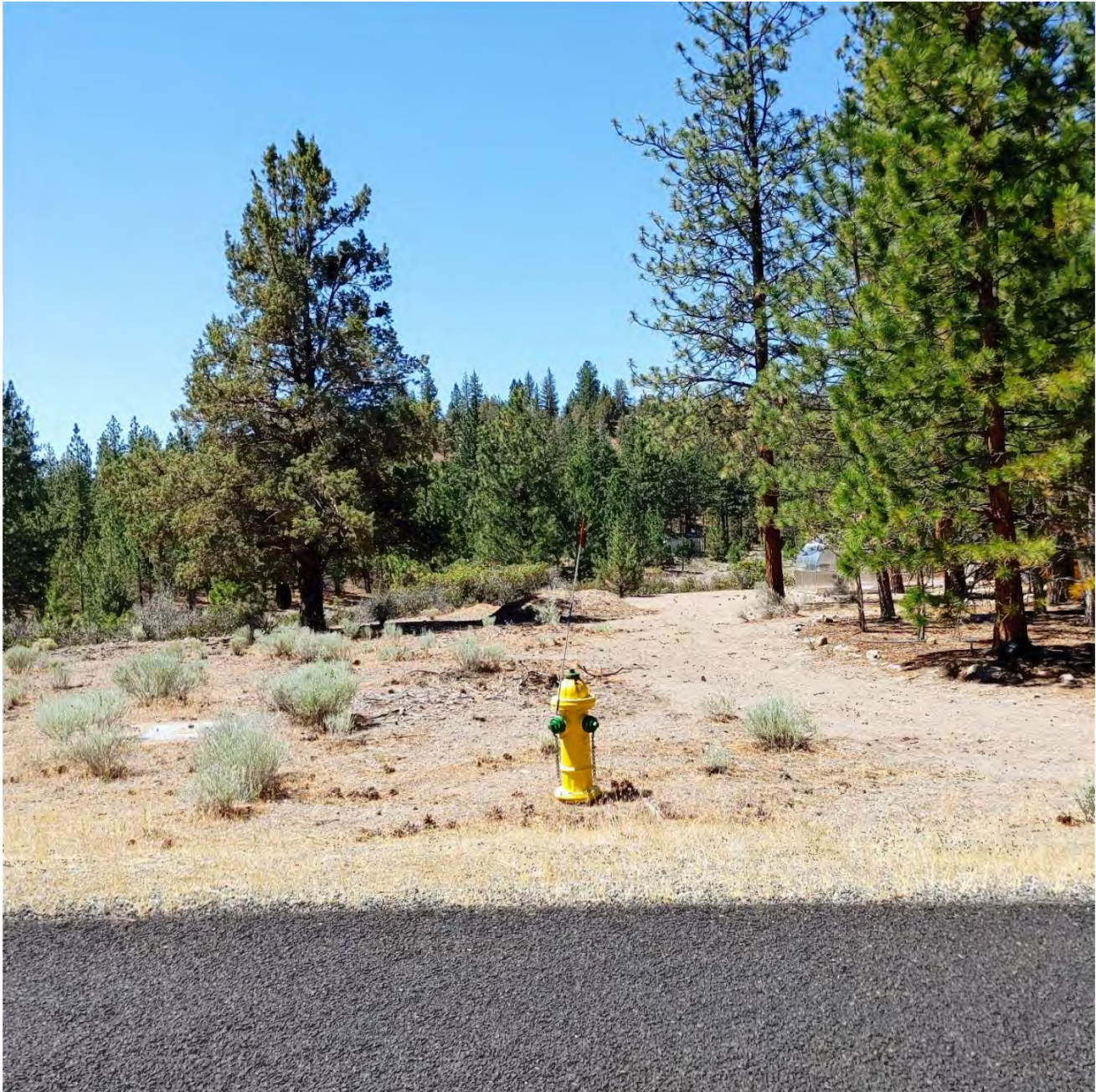
Photo 9: Looking south west from Indian Island onto fire hydrant #79 that will be replaced with a new fire hydrant. This fire hydrant is surrounded by small rabbit brush, gravelly soil, ponderosa pine, and juniper. The soil directly around the fire hydrant will be disturbed as all parts of the hydrant will be replaced down to the elbow in the ground.
