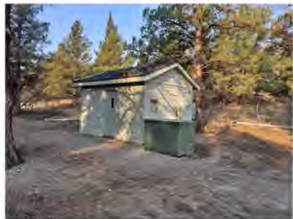
Photograph 3.3 Well #9 Well House
