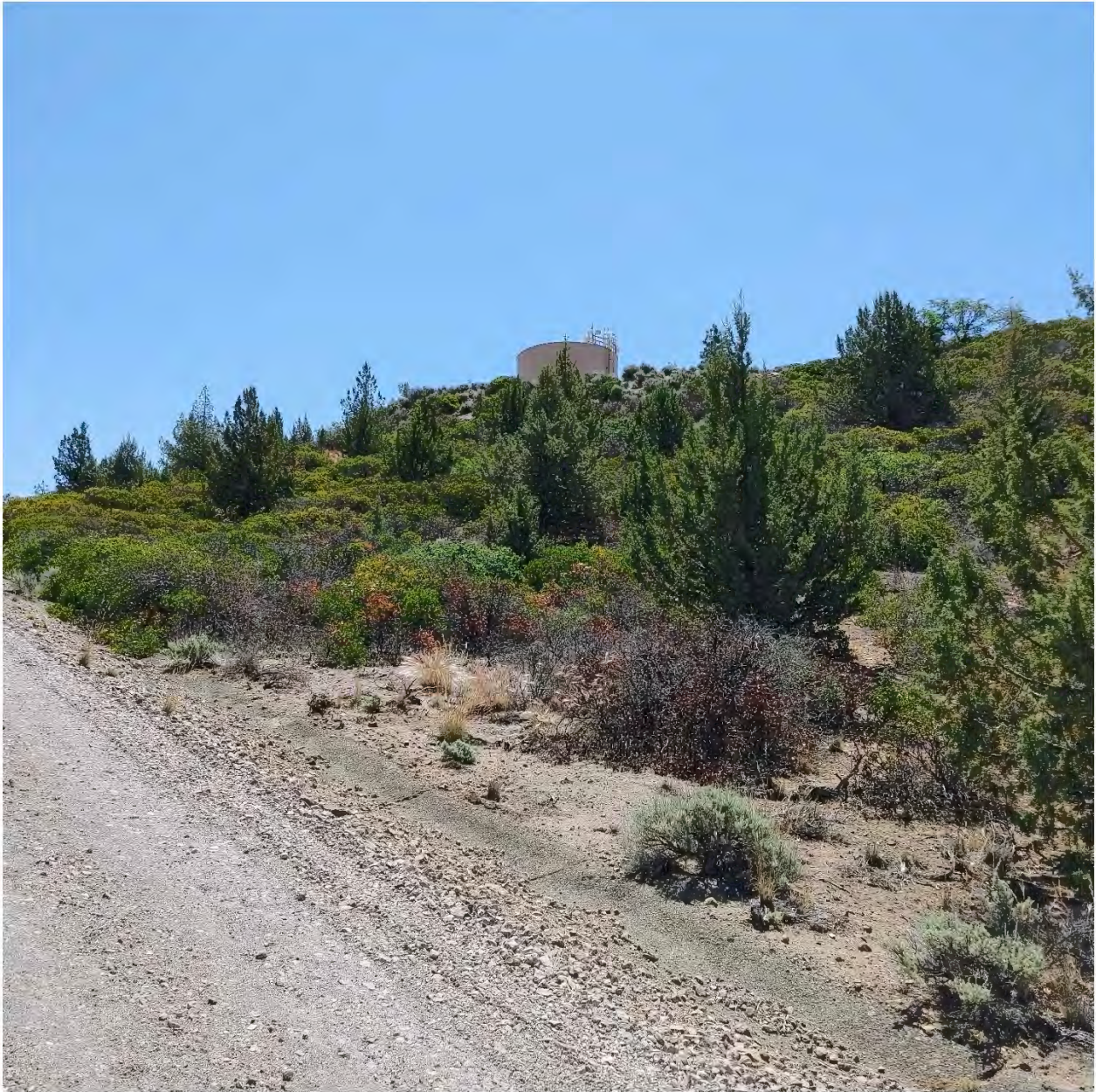
Photo 4: Looking south from the service road to water tank #4 that will be replaced with a larger water tank. Water tank #4 is surrounded by manzanita shrub, gravelly soil, and juniper.
