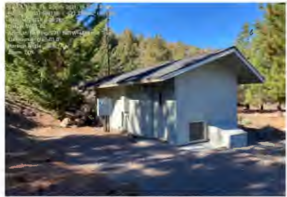
Photograph 3.11 Booster Station B-53
