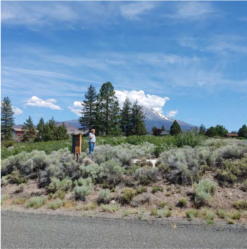
Photo 10: Looking East from Elk Trail Road. Abandoned Pump Station #52 (Figure 3) that is proposed to be a new pump station. The concrete slab that is still present is surrounded by rabbitbrush and manzanita shrub. The soil directly around the concrete will be disturbed when building the pump house. Fire hydrant #190 is the closest to this proposed area (Figure 4).
