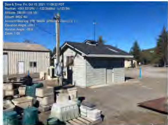
Photograph 3.2 Well #3 Well House
