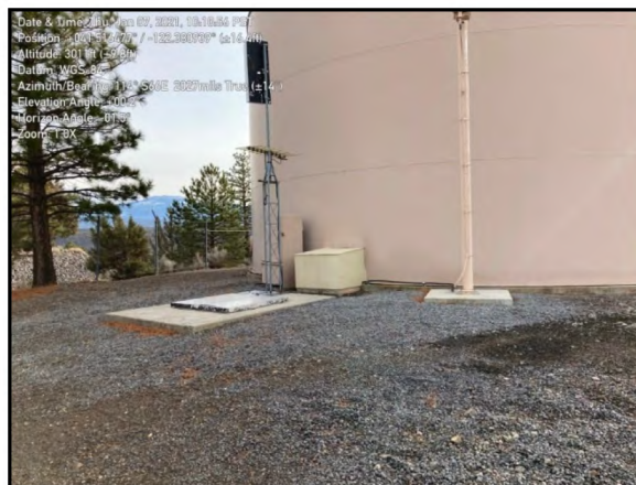
Photograph 3.5 Stag Tank (Tank 2).
