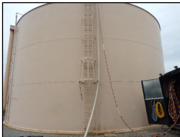
Photograph 3.6 Rancho Tank (Tank 3).
