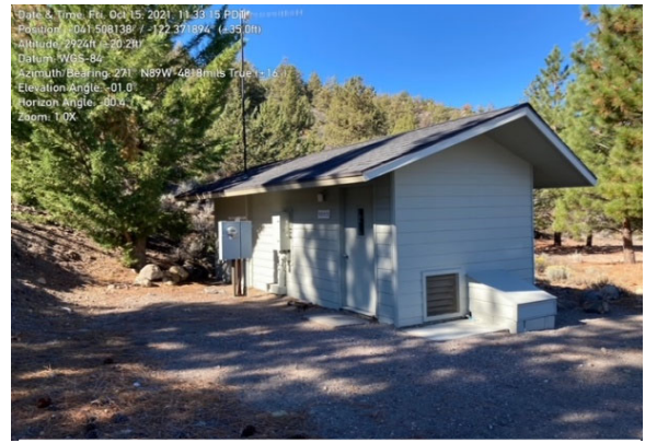
Photograph 3.11 Booster Station B-53
