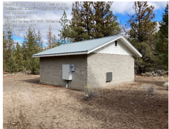
Photograph 3.12 Filling Station B-57
