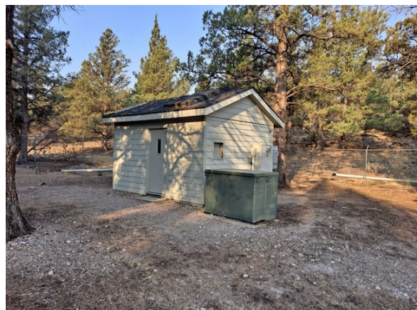
Photograph 3.3 Well #9 Well House
