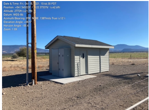
Photograph 3.1 Well #4 Well House
