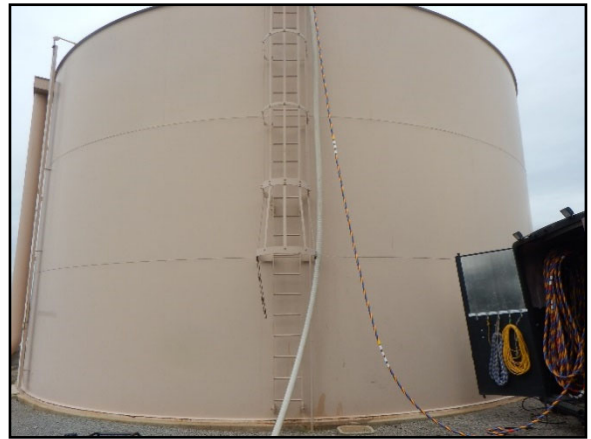
Photograph 3.6 Rancho Tank (Tank 3).
