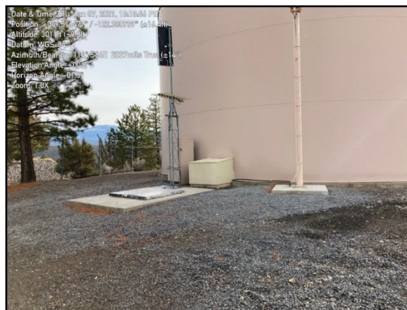
Photograph 3.5 Stag Tank (Tank 2).
