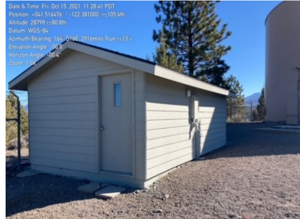
Photograph 3.9 Booster Pump Station B-51
