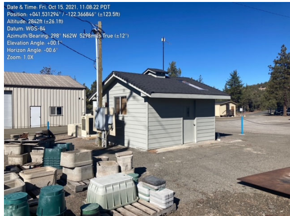
Photograph 3.2 Well #3 Well House
