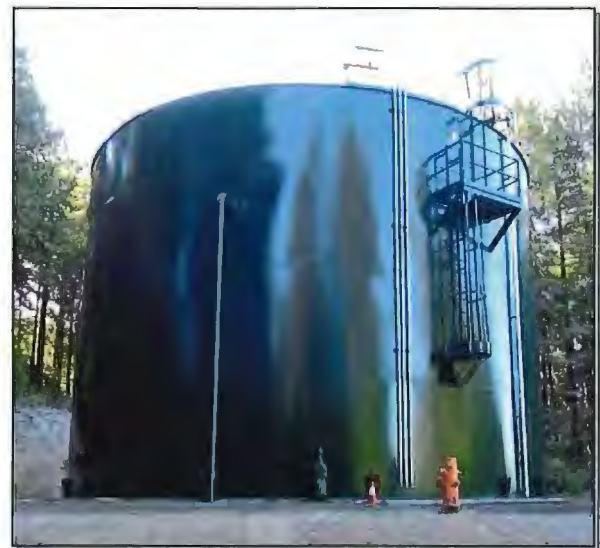
The City of Arcata's new Upper Panorama tank (welded steel).
