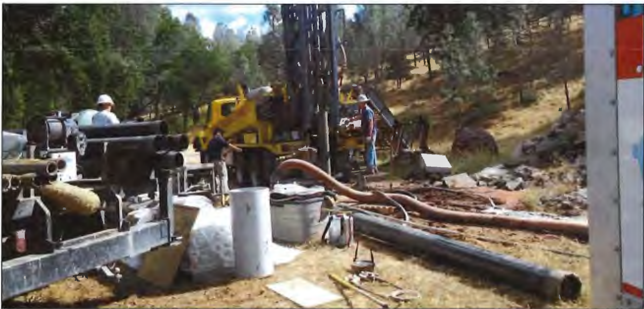
SHN supervised the well installation activities at CAL FIRE's Ishi Conservation Camp in Tehama County. The project included installation of two wells and a pair of 10-day pumping tests, complex permitting, and an aggressive schedule.
